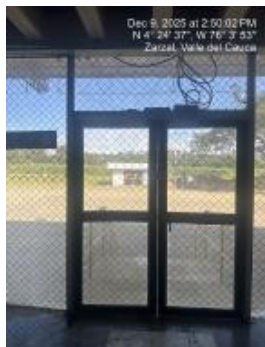
Emergency Exit (2).JPG
