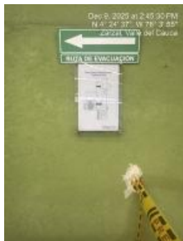
Evacuation Route Signage.JPG
